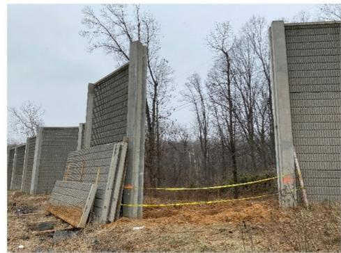
*Noise wall panels removed to provide access for boring rigs along southbound I-495 between Georgetown Pike and Old Dominion Drive.*
