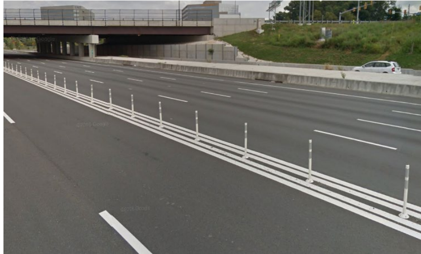
Figure 2-1. Existing Flexible Post Delineators on I-495 Express Lanes
